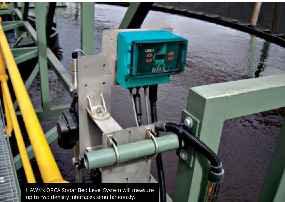
HAWK's ORCA Sonar System shown in a thickener application
