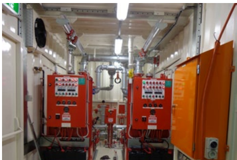
Kelair's fully packaged fire pumpsets are factory tested as a complete assembly to the requirements of ISO9906 Grade 1U and AS2941.
