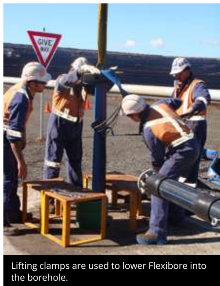
The installation was completed using a crane and lifting clamps.
