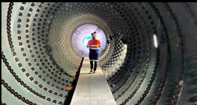
(Image source: Albemarle) A worker inspects shotcrete refractory work during construction of lithium processing trains 1 and 2 at Albemarle's Kemerton lithium hydroxide processing plant near Bunbury, WA. The image shows the feed end of the calcine kiln, along with chain cleats on the internal wall, prior to chain installation.
