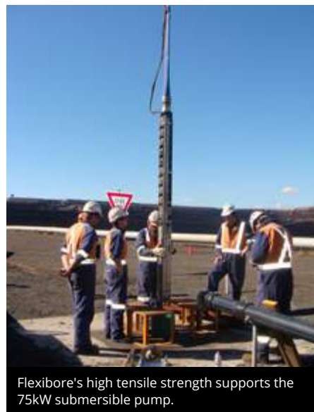
The installation was completed using a crane and lifting clamps.
