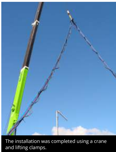
Flexibore's high tensile strength supports the 75kW submersible pump.
