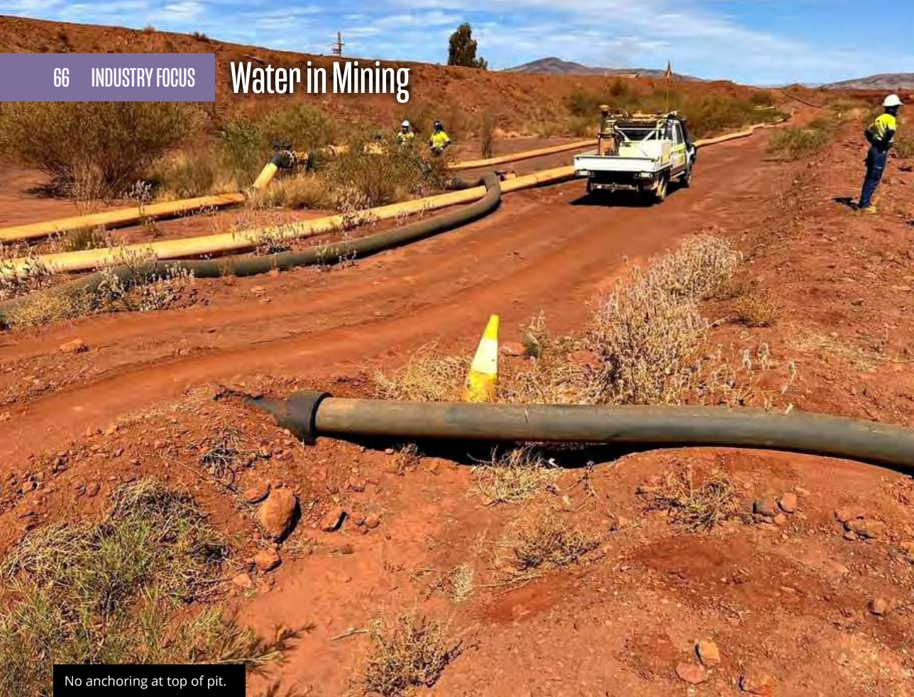
Layflat pipeline connected to the ring main.
