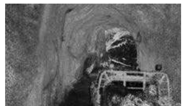
A point cloud from a rapid scan carried out with the handheld Zeb Horizon identifying rock structures before shotcrete and mesh was installed.
