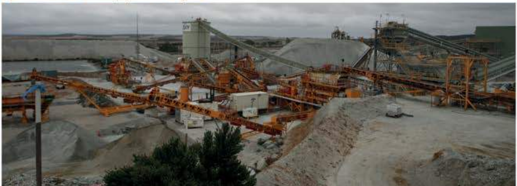
Rapid's extensive circuit with Galaxy's plant in the background
