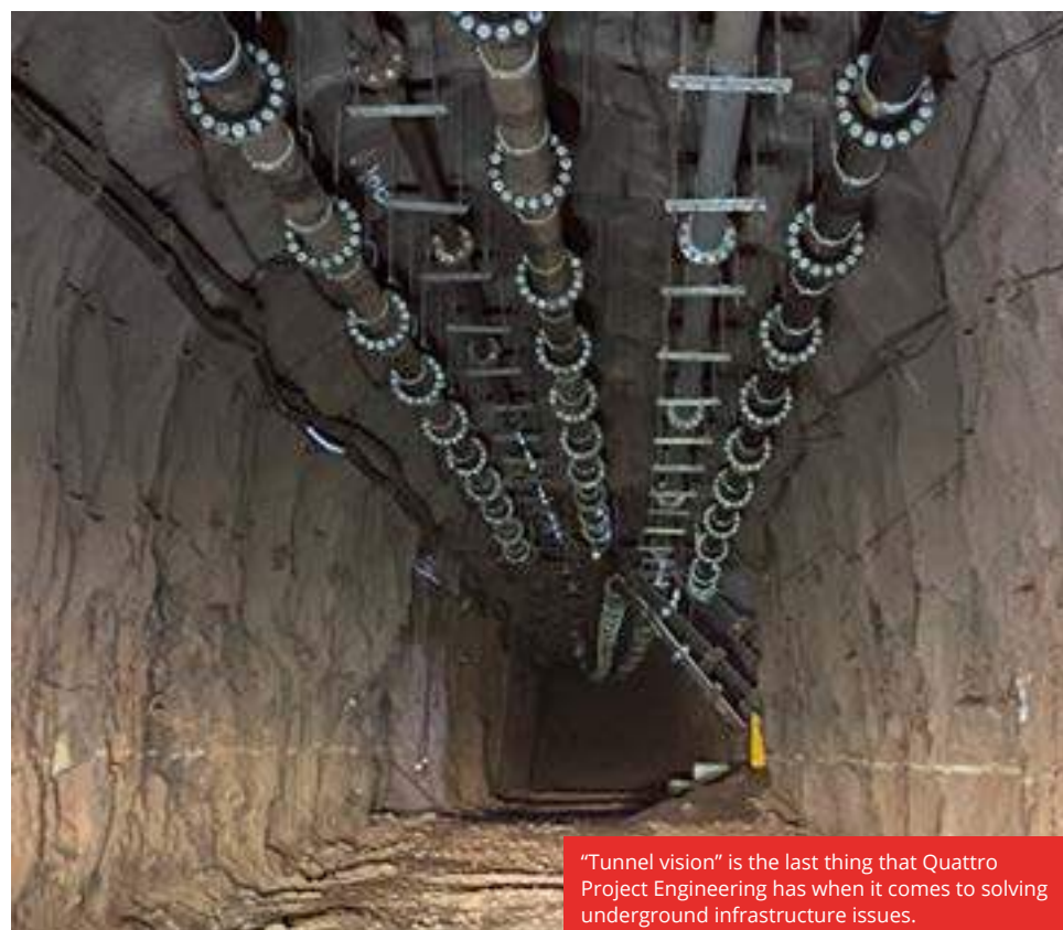
The QBrace interfaces with the hanging fastener of the QClaw, with strut arms cut to length then secured to the backs via rock bolts, creating a certified, tensile bracing system that resolves loads to rock.
