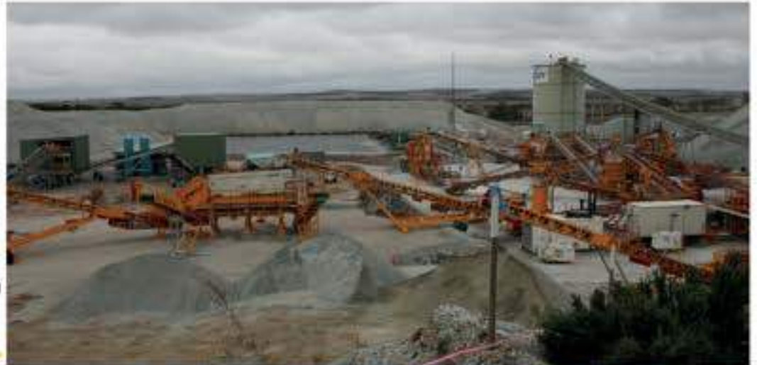
Rapid's circuit in the foreground servicing Galaxy's Optical Ore Sorting plant in the background left.
