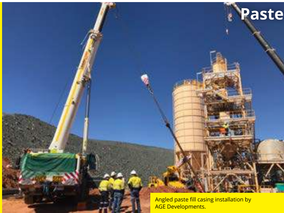
Paste fill casing is installed/removed utilising AGE's hydraulic tong equipment.
