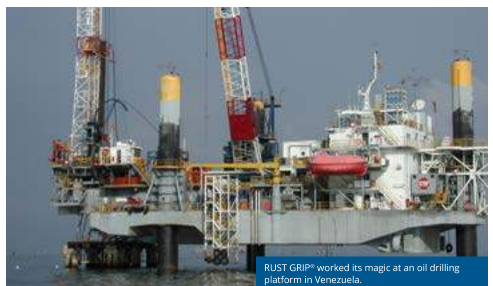
Mitsubishi's 'tank terminal' in Japan was coated with SUPER THERM® to stabilise fuel and oil storage.
